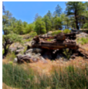
Old Rail Trestle
